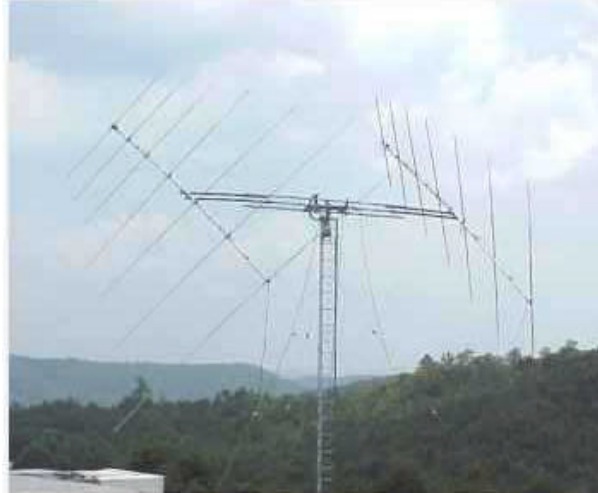
PARI's pair of M-Squared 17-30LP7 log periodic yagis for Jupiter/Io and Solar Observations
